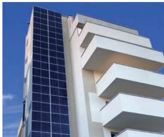
PANNELLI SOLARI INSTALLATI IN FACCIATA CON SISTEMA DI FISSAGGIO TEKNOMEGA
